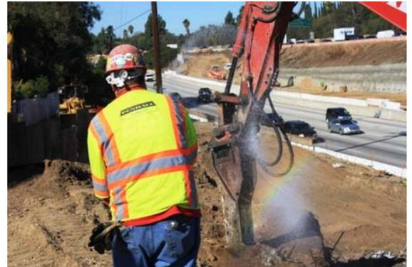
A member of the construction team sprays water on a large impact drill creating a rainbow as it demolishes the old bridge abutments.
